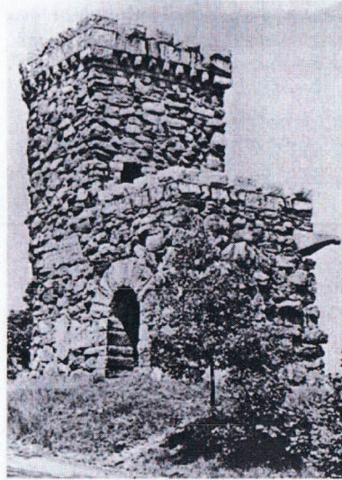
This is the 1889 Davis Tower at Worcester, Mass., upon which was hung a tiny plaque in 1910 honoring Samuel (Leonardson) Lenorson, the boy who helped Hannah Duston flee Indian captors in 1697. The tower was demolished two years ago because of disrepair and the tablet disappeared four years ago. The Worcester Historical Society has a plaster cast of the tablet. — Photo by Worcester Telegram & Gazette.
