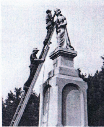
Workmen of the John Swenson Granite Co., of Concord are shown patching Hannah Duston's nose, and other vandalism scars. Robert C. Sampson did the surgery with granite dust, assisted by Emanuel Brochu.
